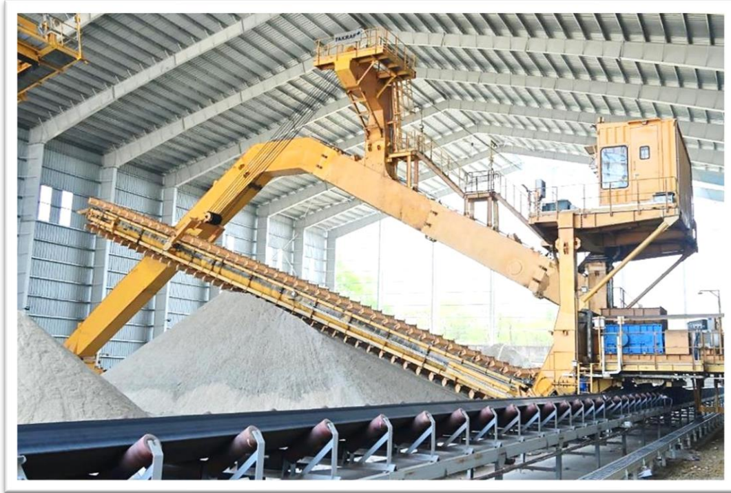
Stacker Reclaimer and Shed
