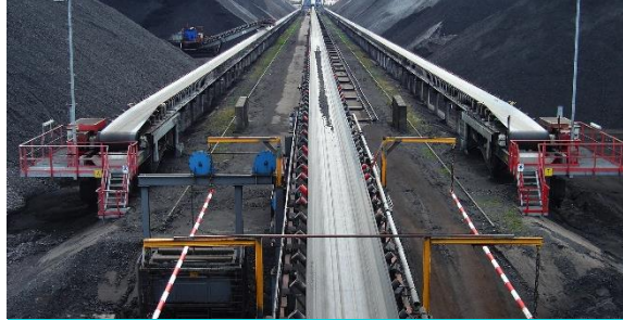
Coal Mine Railway Conveyor Belt, Maharashtra
