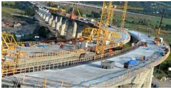
Bangalore-Chennai Expressway one of the 26 new green expressways
